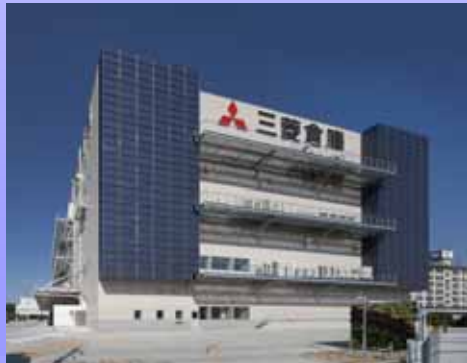
[Ibaraki Warehouse #3/ Osaka]
