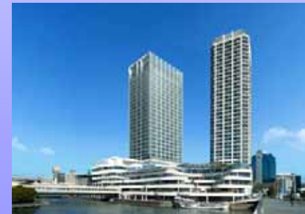
[Yokohama Dia Building]
