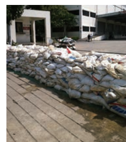
Piling up bagged sand to address possible submergence
