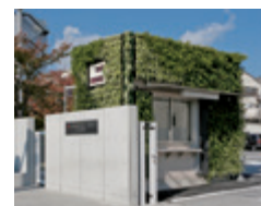
Greening of the rooftop and wall surfaces of the guard's station at Ibaraki Warehouse No. 3
