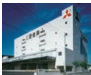
Kinjoh Warehouse, Nagoya Branch
