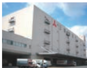
Aomi Distribution Center No. 1, Tokyo Branch
