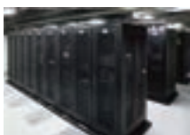
Disaster countermeasure center in the Kansai region
