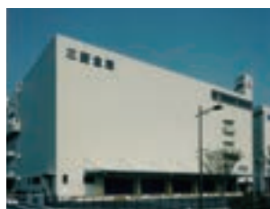
Chuo Futo Warehouse, Fukuoka Branch
