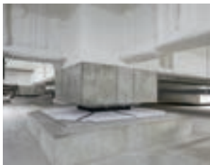
Seismic isolation rubber and seismic isolation dampers (Misato Distribution Center No. 2 Phase 2 building, Tokyo)
