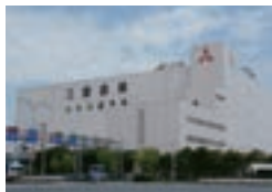
1999 Automated warehouse (Ohi Refrigerated Warehouse)
