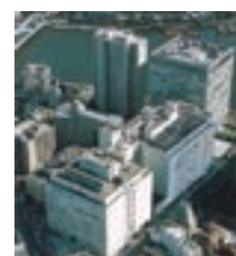
1973 Tokyo Dia Building
